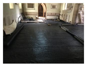
The whole of the floor in the Nave, North Aisle and the South Transept has now been levelled, the geotech membrane is in position and the net to which the heating pipes will be fixed has been laid throughout, apart from over the 'Pool' vault, which will have a thin layer of screed and the stone surface on top. The architect is still in discussion with Westford Mechanical, the heating engineers,
