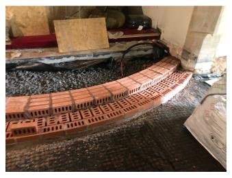
stone steps, in a curve, on top. There will be under-floor heating in the Chancel, but not in the Sanctuary, instead there will be a radiator on the wall on each side on the same heating circuit as the under-floor heating in this area.
